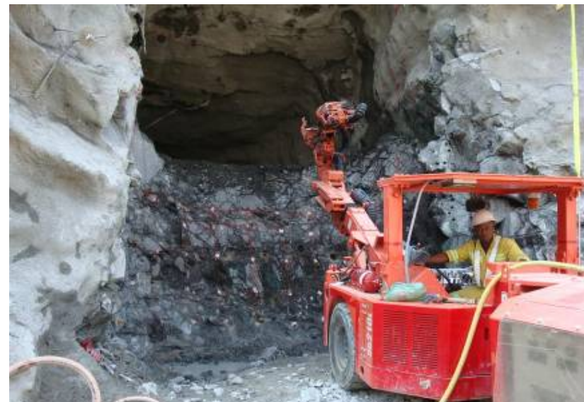
Decline shaft development at Eland
