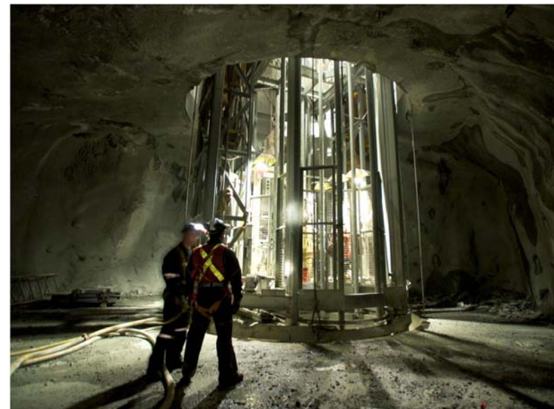
Shaft sinking at Nickel Rim South
