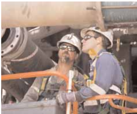
Maintenance crew works on the concentrator plant at McArthur River Mine
