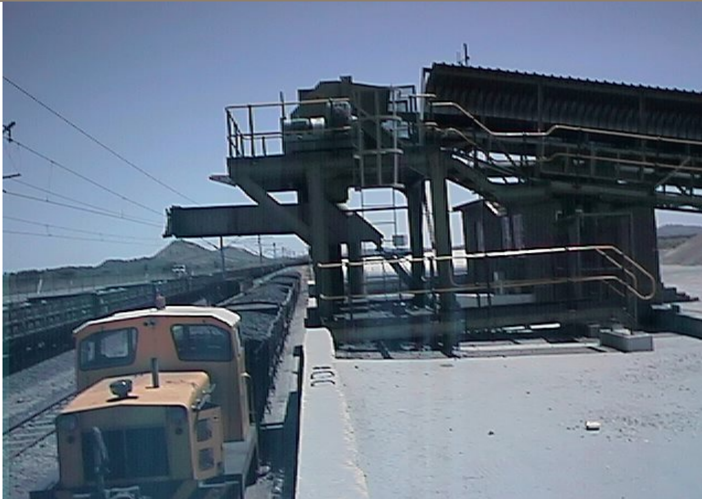
Final load and sampling station for sized product rail loading
