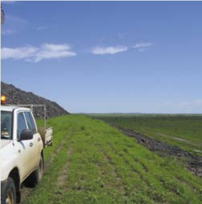
South West Tier 1 Rehabilitation completed in September 2005 primarily made up of Mitchell and Flinders Grass.
