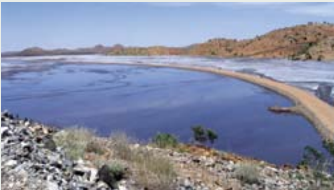
Mount Isa Mines tailings management system.
