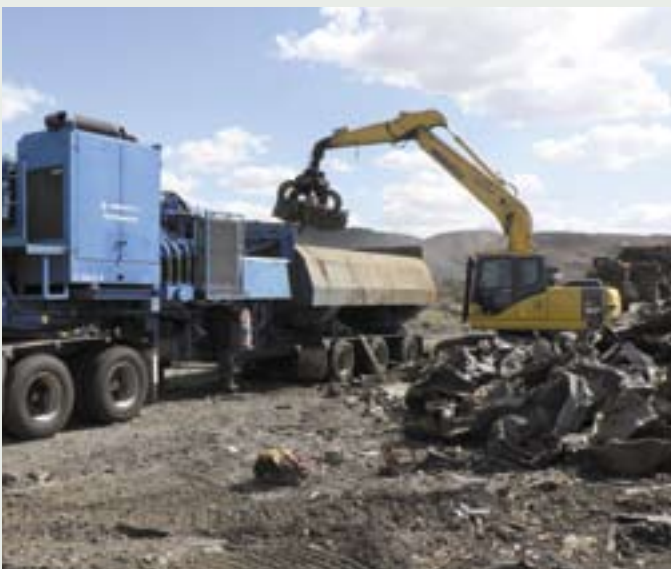
Light gauge scrap metal being compacted into bales for transport to the recycling facility.
