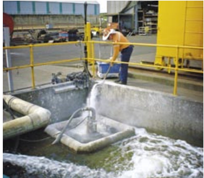
Senior Operator Bob Griffin takes water samples from a sump at the Townsville Port. In 2004 Xstrata upgraded its environmental monitoring system at the port and undertook a major capital works program to ensure contaminants were not escaping from the operations into the environment.
