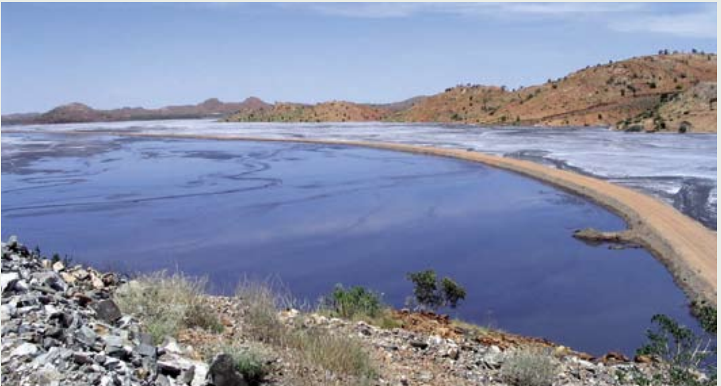
Mount Isa Mines tailings management system.
