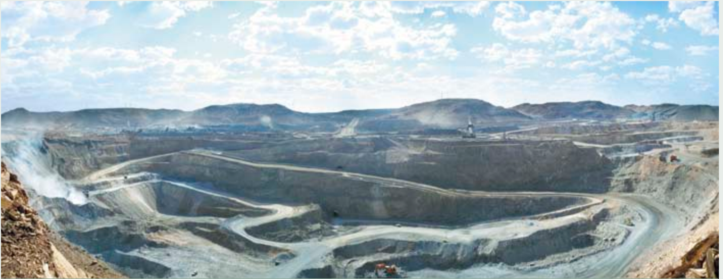
Black Star Open Cut pit. Environmental Advisors are heavily involved in correct handling of waste rock from the pit and in controlling dust generation.
