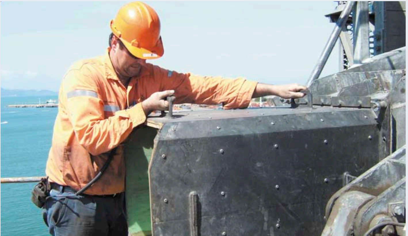
Peter Smith fits the gimble chute, an innovation from the Townsville Port employees.
