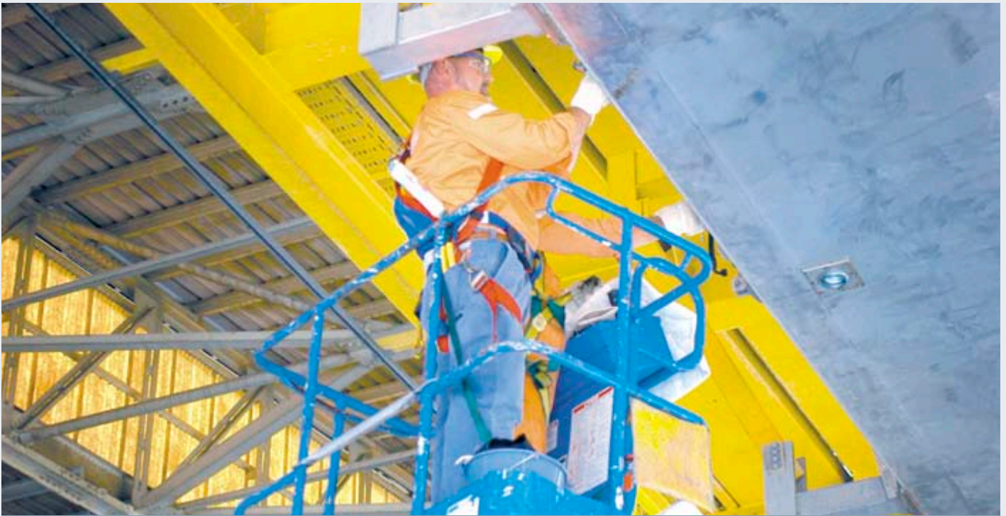
Trades Assistant Maintenance, Steve Jensen, undertaking maintenance on the refinery crane.
