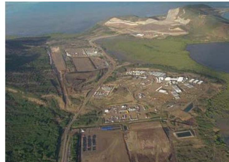
Site establishment and earthworks in New Caledonia
