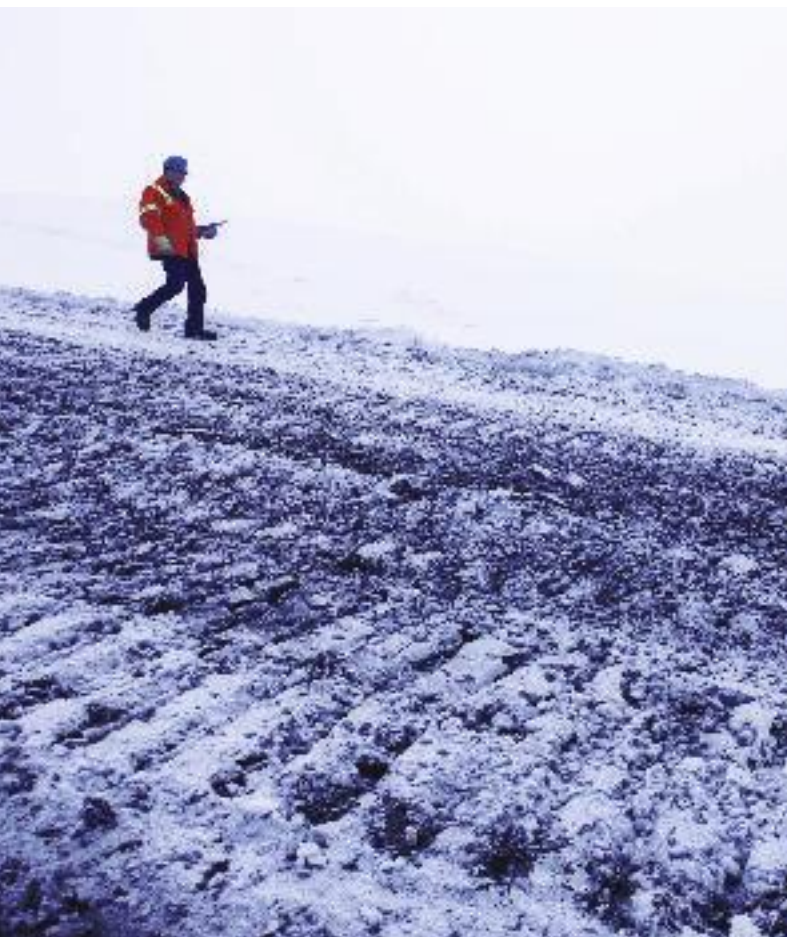
Sylvain Pomerleau inspects the tailings dam at Xstrata Nickel's Raglan mine.
