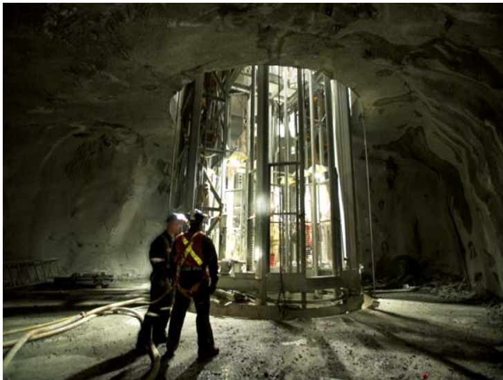
Photo: Nickel Rim shaft sinking
