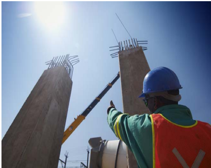
Photo: Goedgevonden railway siding construction
