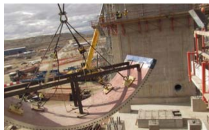
Sag Mill mounting at Antapaccay
